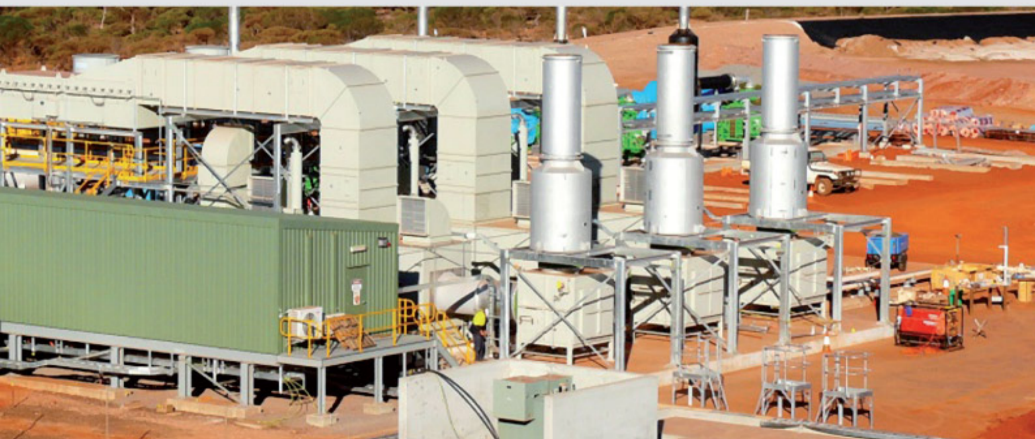
Opposite page: Welder in Pipe Above: Gas Turbine installation Windimurra
