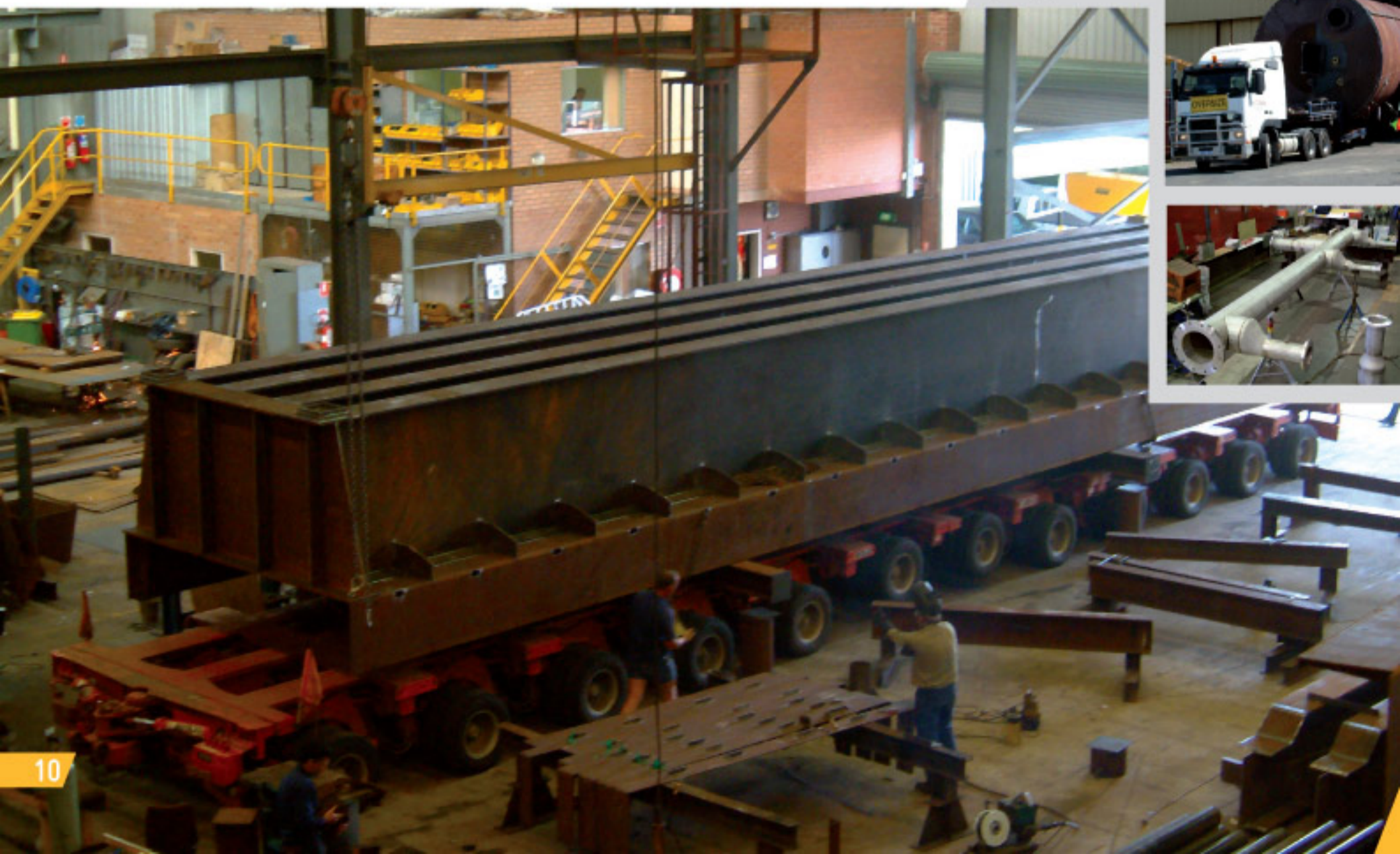
Below: Railway bridge fabrication
