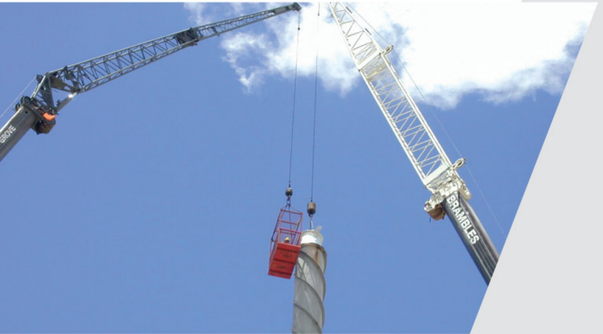
Above: Odour reduction Stack
